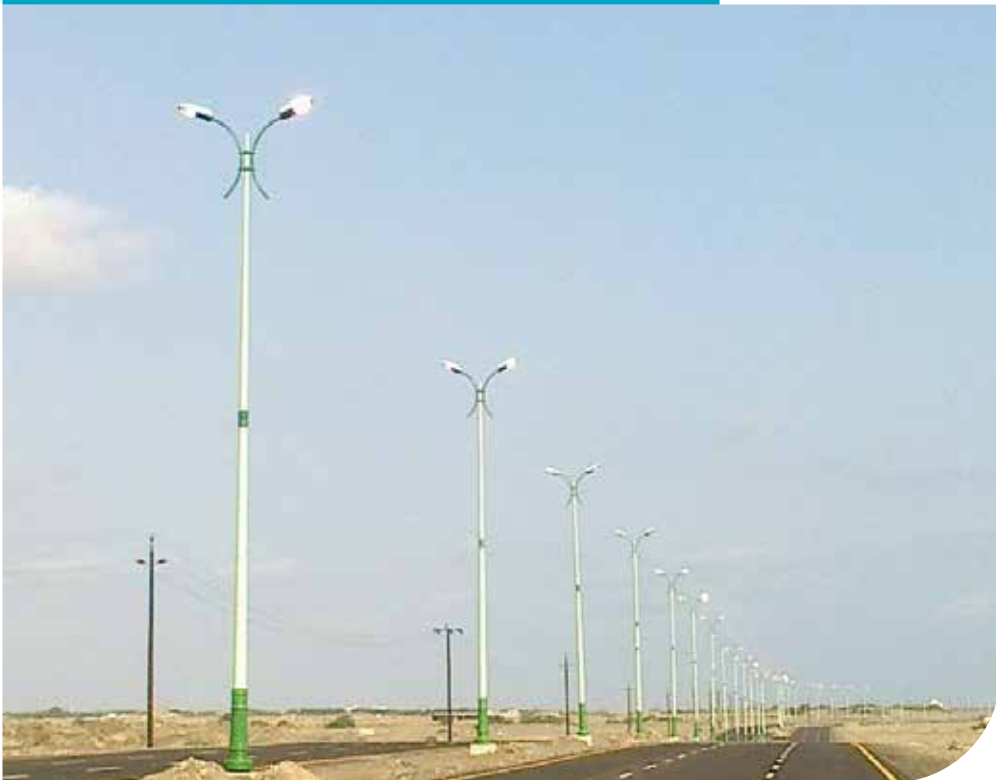
Zanjibar Road - Yemen
