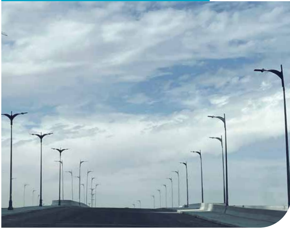
Street Lighting Poles
